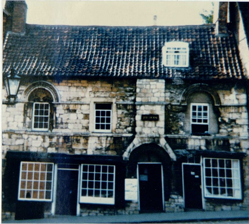
Belasset's House now No.8 Steep Hill Lincoln.
